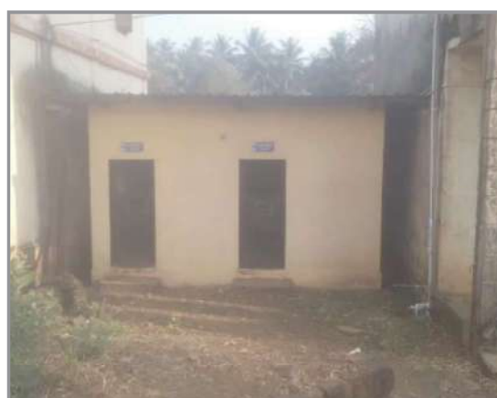
Toilet construction in the school
